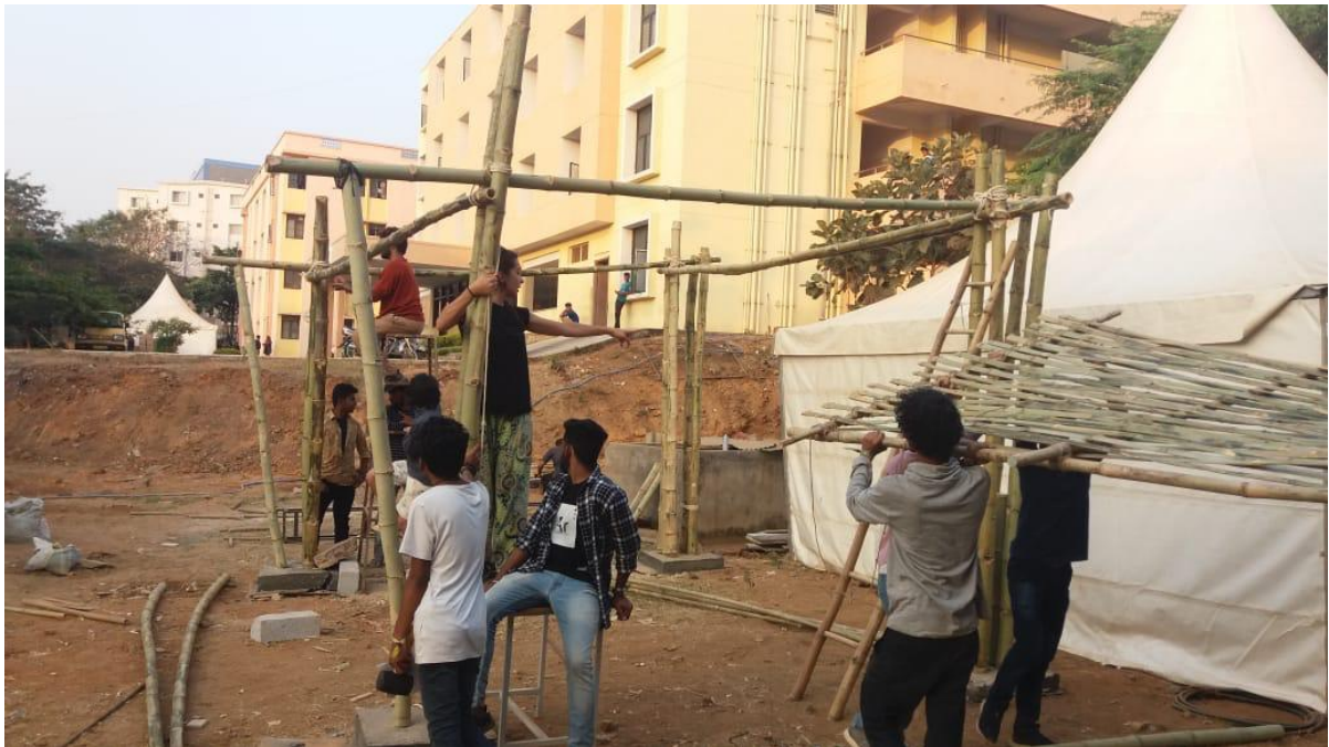
Fig. 5: One of the bamboo structures under construction
