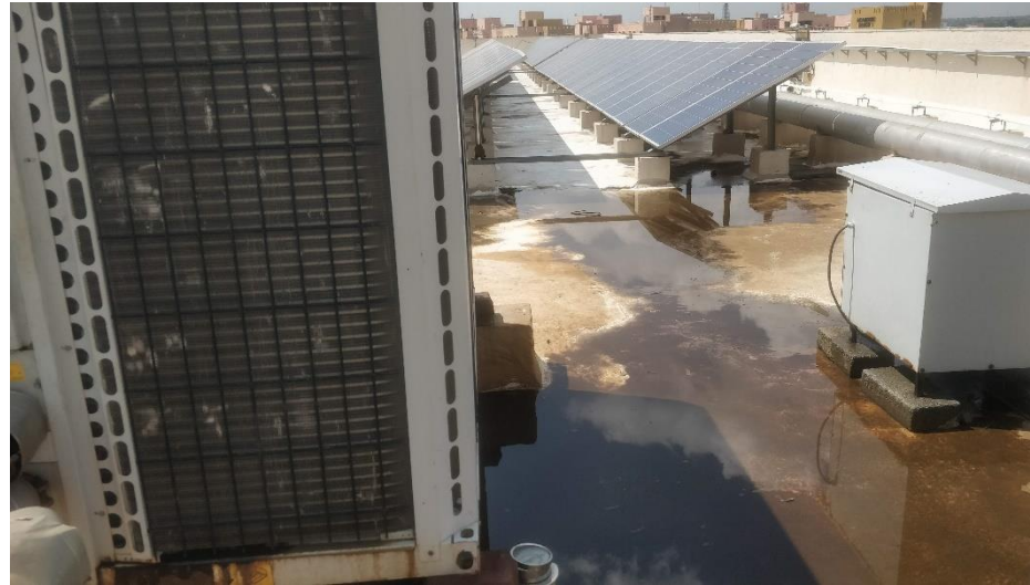
Image 6: Leakages in chiller supply and return water lines
