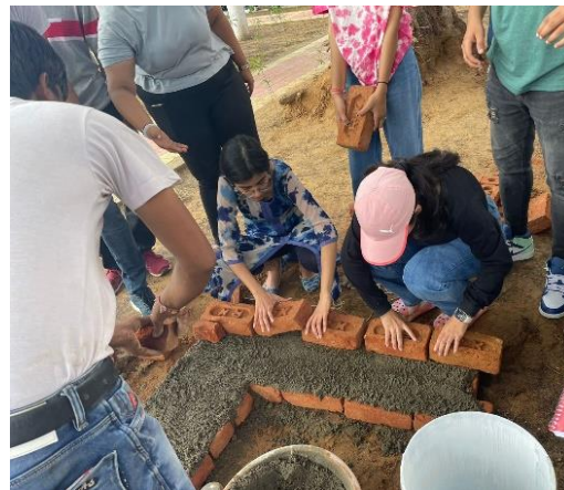
Brick bond preparation by Students in Workshop
